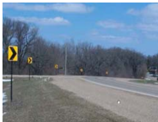
Freeborn County, MN Installed chevrons along horizontal curves
