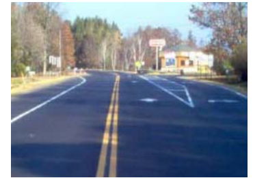
Crow Wing County, MN Installed offset turn lane
