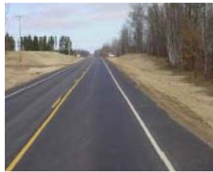
Cass County, MN - Paved shoulders and improved right way
